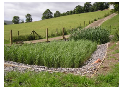
Example of a reed bed system
